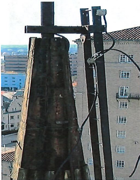
Copper removed at top of steeple. Large cables visible attached to lightning rod
