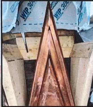
THE TEAM ALSO WORKED ON RESTORING EXISTING WOODEN STRUCTURES, CLADDING THEM WITH COPPER.
