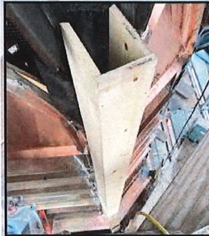
THE TEAM ALSO ATTACHED THE REPLACEMENT COPPER CLADDING TO THE MAIN STRUCTURE
