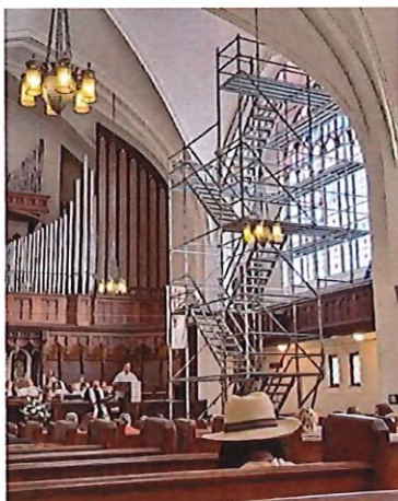
Restoration work in progress on a side aisle window.
